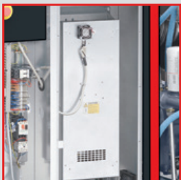
Frequency converter
